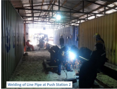
Welding of Line Pipe at Push Station 2
