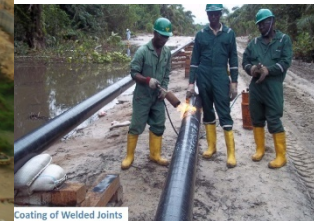
Coating of Welded Joints
