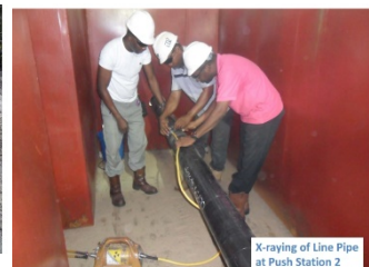
Kraying of Line Pipe at Push Station 2
